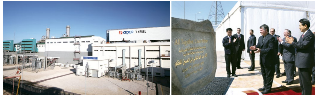
KEPCO's first IPP project in the Middle East, Al Qatrana IGCC Power Plant (373MW), provides 12% of Jordan's electricity.
