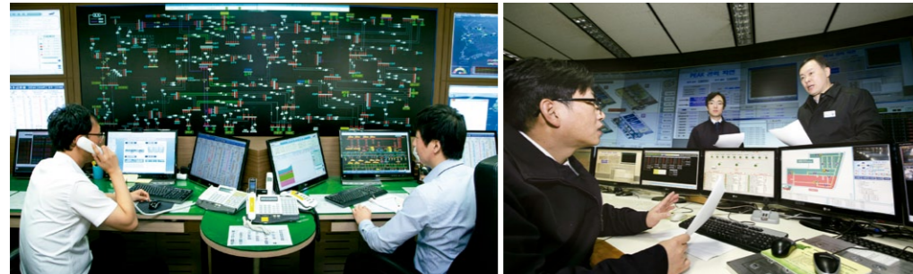
KEPCO operates a 24/7 emergency response system to maintain stable power supply.
